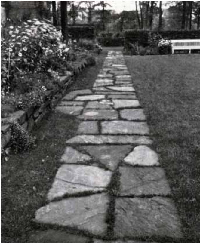
■ Slab path with grass joints. The stone path is interrupted with some kind of vegetation, here grass. (Poethig, Kurt & Camillo Schneider 1929 Hausgartentechnik , Berlin-Westend, p. 47)
